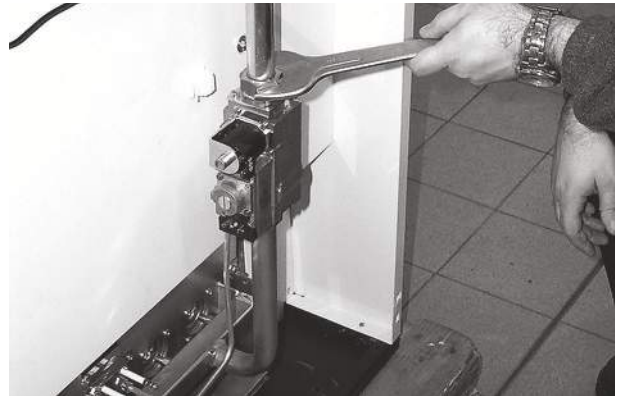
fig. 9 - Undo the gas valve nut
